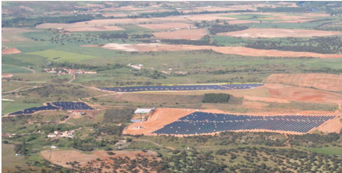
Planta Solar de Salamanca consists of three solar arrays on a 36-hectare (89-acre) site.
